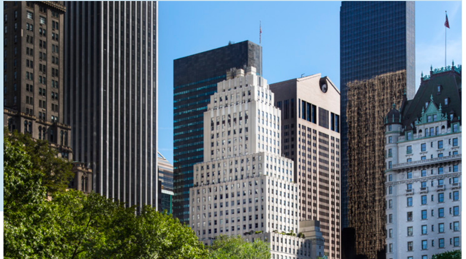
View of 745 Fifth Avenue (NY) from Central Park
